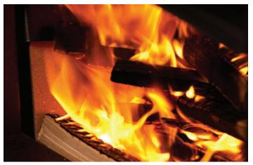
**15 Minutes -** Blower shuts down. Homeowner adjusts damper and air controls to maintain fire.
